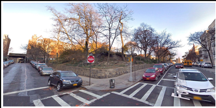
Retaining walls at Bennett Park's southeast corner (Fort Washington Avenue & West 183rd Street) [screen-capture from Google Maps/Street View]
